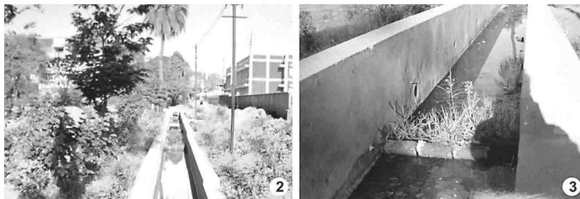
Figs 2-3. The open drain as seen from the eastern end, showing the accumulated water due to the presence of single brick layer placed across its floor at regular intervals: (2) the north wall in shade; – (3) the well-lit south wall of the drain.
